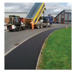
New constructions require good quality, non-plastic, well compacted sub-base (i.e. Type 1). Installation should be carried out in accordance with the general requirements of BS 594987, using as large a tandem roller as possible for the site. Pedestrian single-drum rollers and wacker plates should only be used in areas of restricted access, and to remove any marks left by the lead roller. The material shall be substantially compacted before reaching 110°C.
